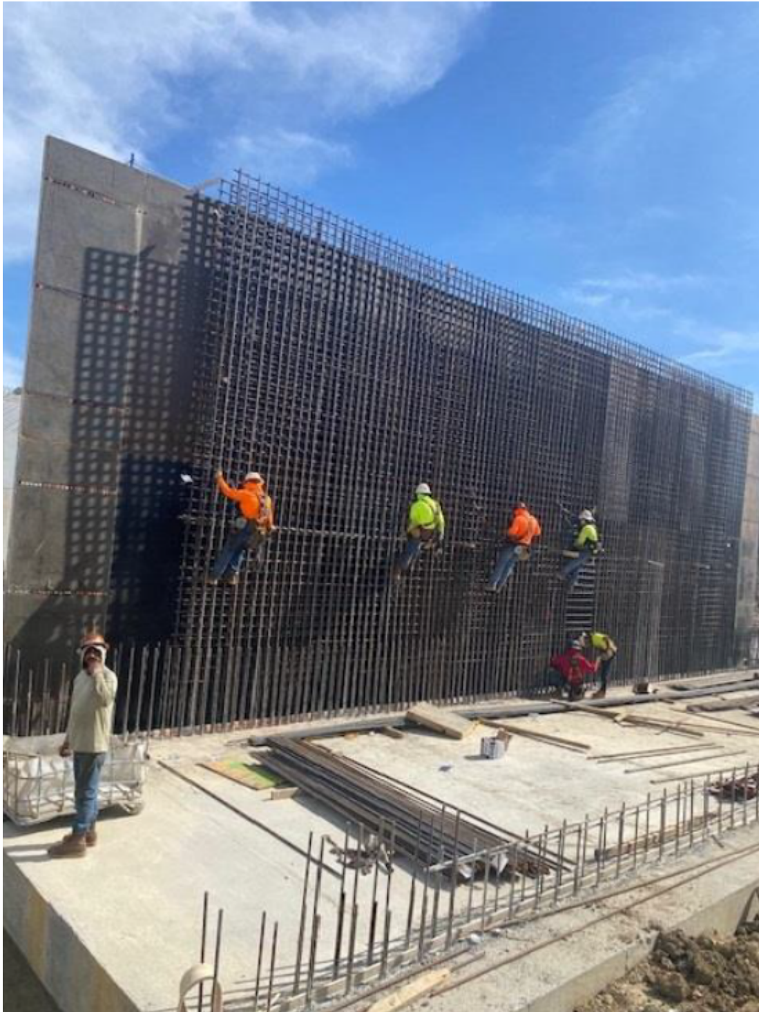
Steel tying on the SBR structure
