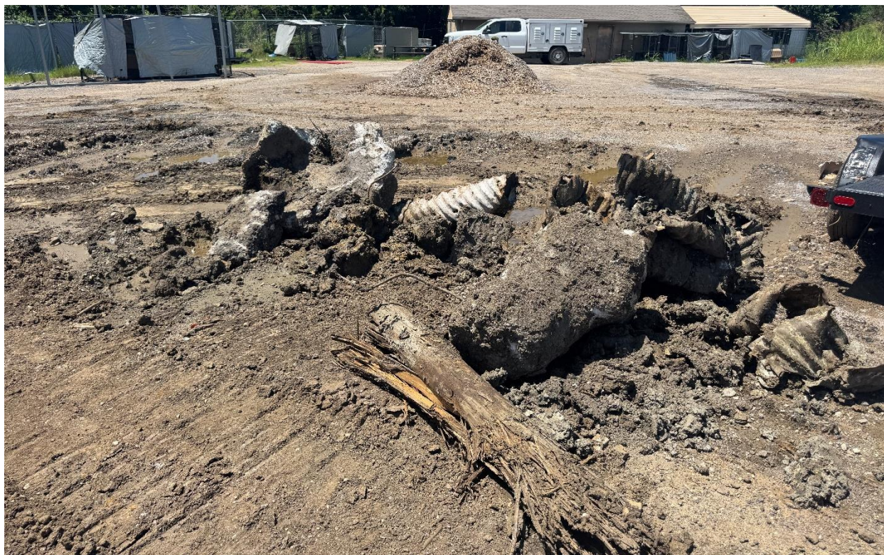
Photograph 4: Corrugated pipe, timber and concrete removed from excavation
