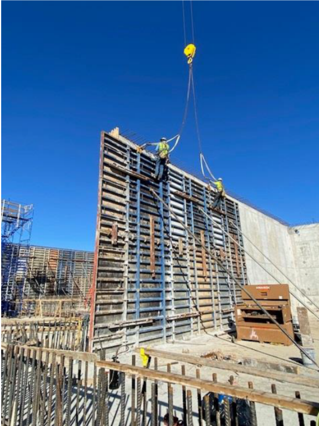
Formwork on the SBR structure
