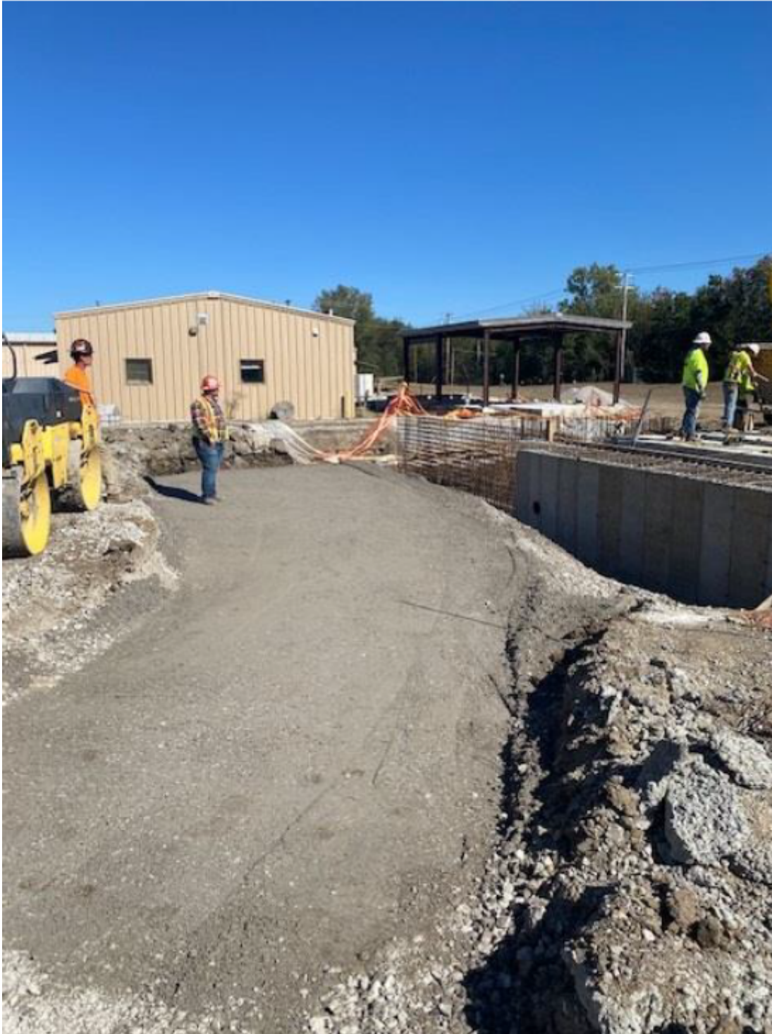
Aggregate base at Headworks structure
