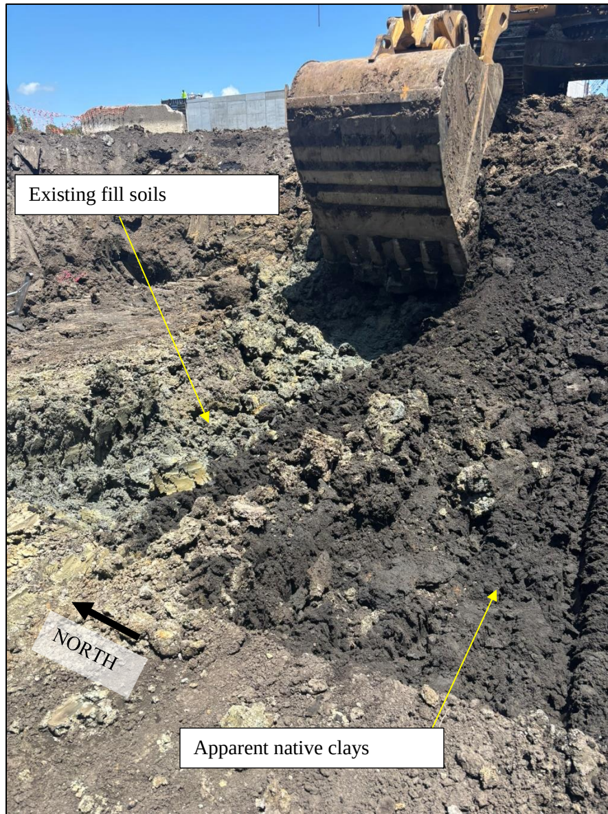
Photograph 2: Test pit at 'upper bench' where exposed soils were roughly at 3 feet below bottom of footing. Test pit exposing existing fill with concrete and asphalt cobbles.
