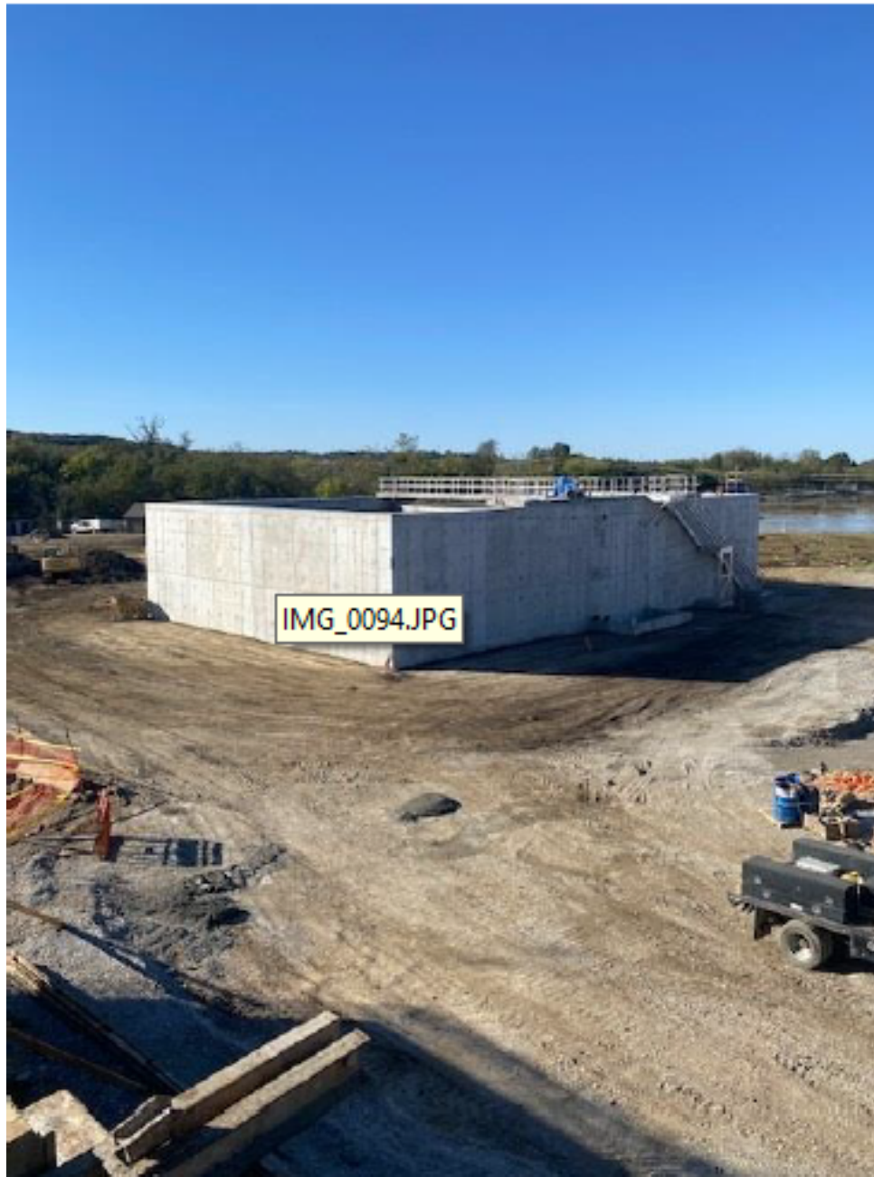
Backfill to south and east wall of the digester
