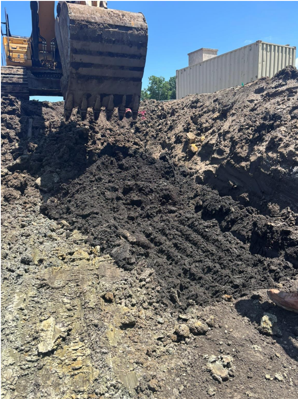
Photograph 6: Presumably native lean clay along the south edge of the excavation at roughly 4 feet below bottom of plan foundation elevation
