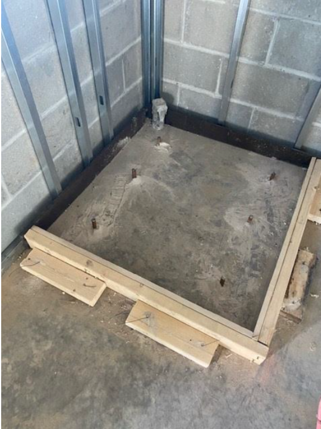
Concrete for Utility pad at the Admin Building
