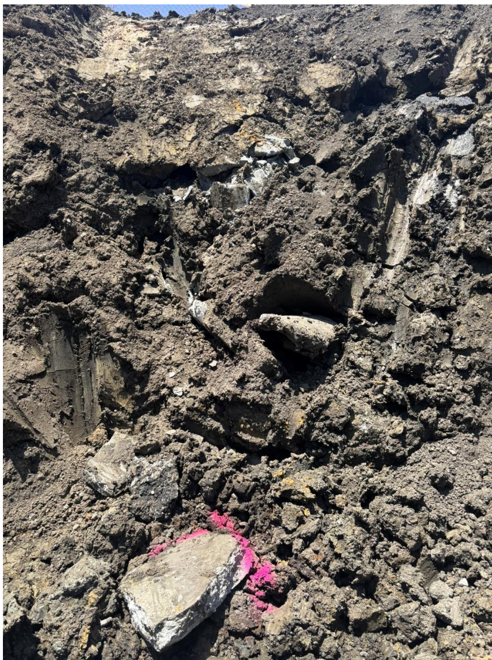
Photograph 5: Northeast corner of excavation with concrete debris in the sidewalls
