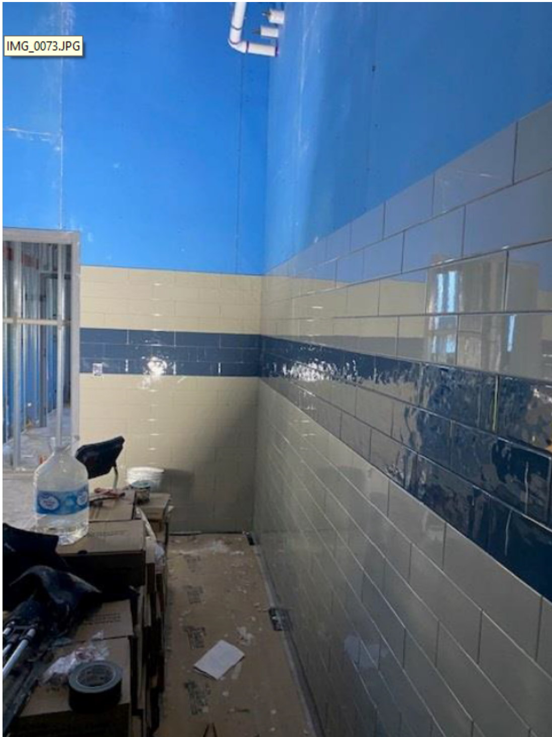
Tile Installation at the Admin Building
