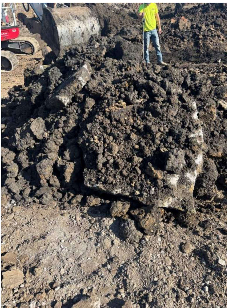
Photograph 1: Existing fill and concrete found at -4.0' below FSG at NE test pit.
