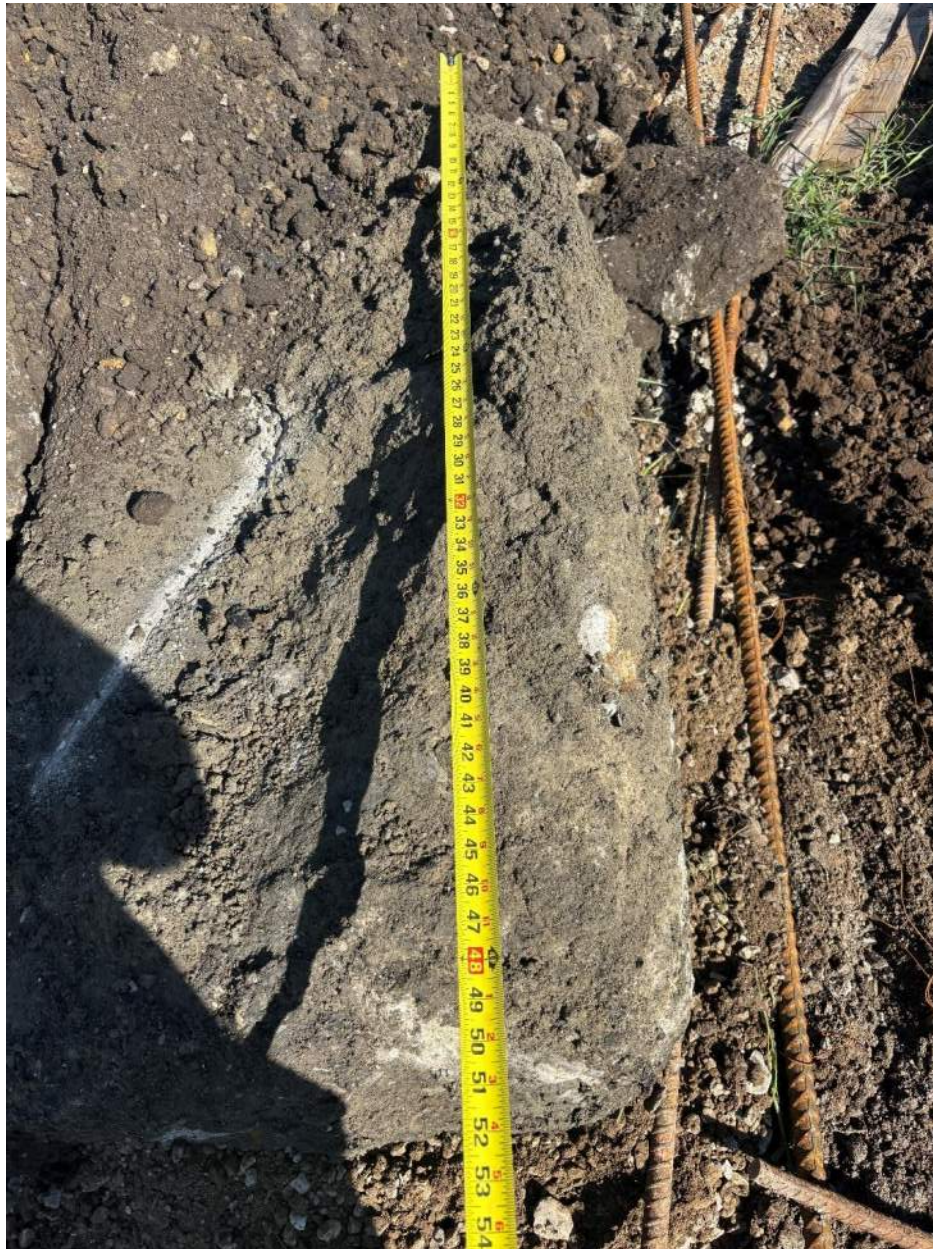
Photograph 10: Concrete slab removed from test pit excavation
