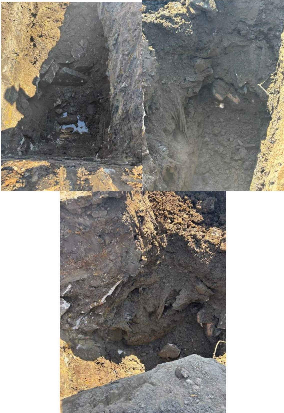
Photograph 5-7: Debris in pits during excavation.
