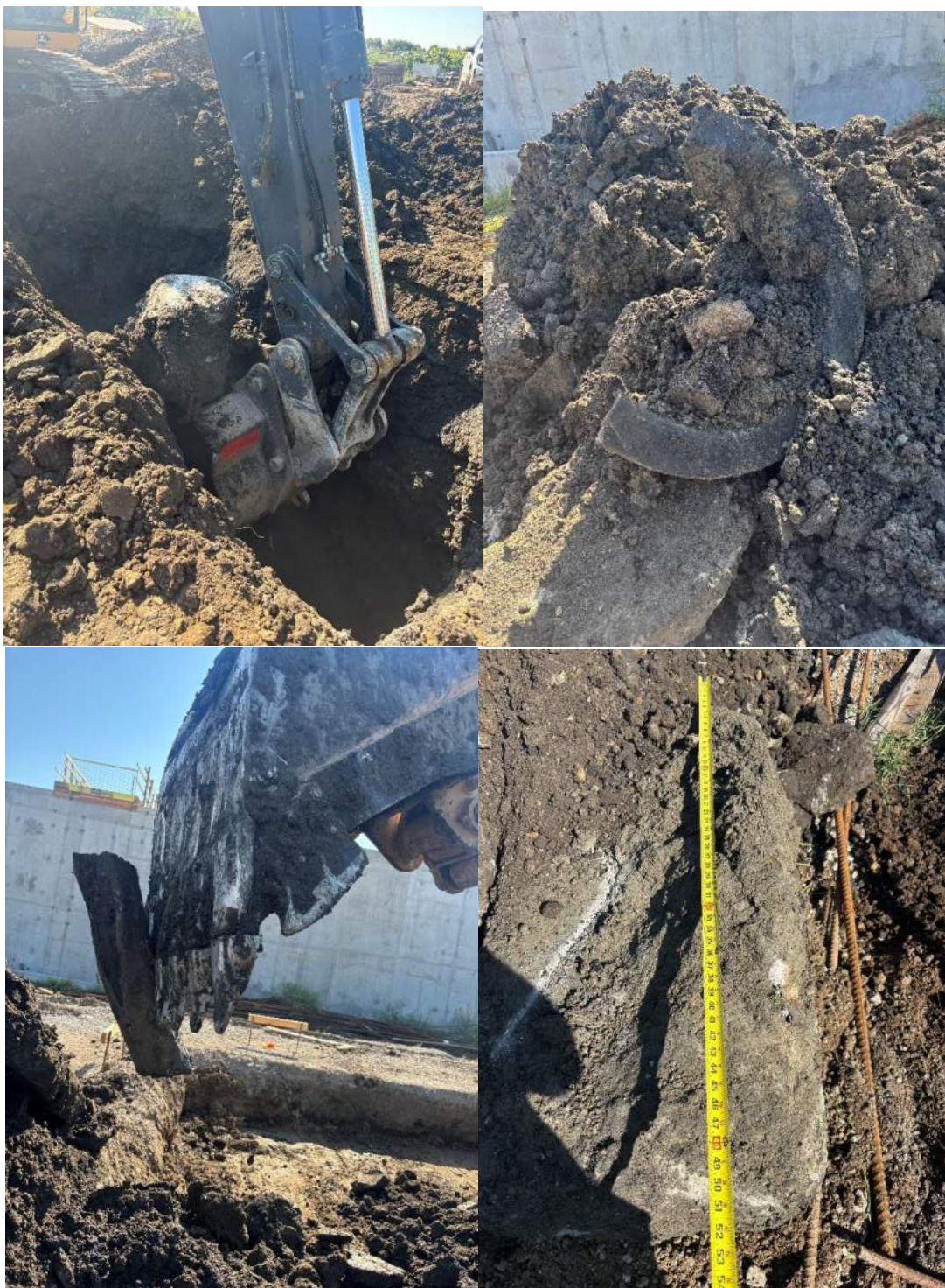
Photograph 2-4: Showing debris removed from excavations from all three pits.
