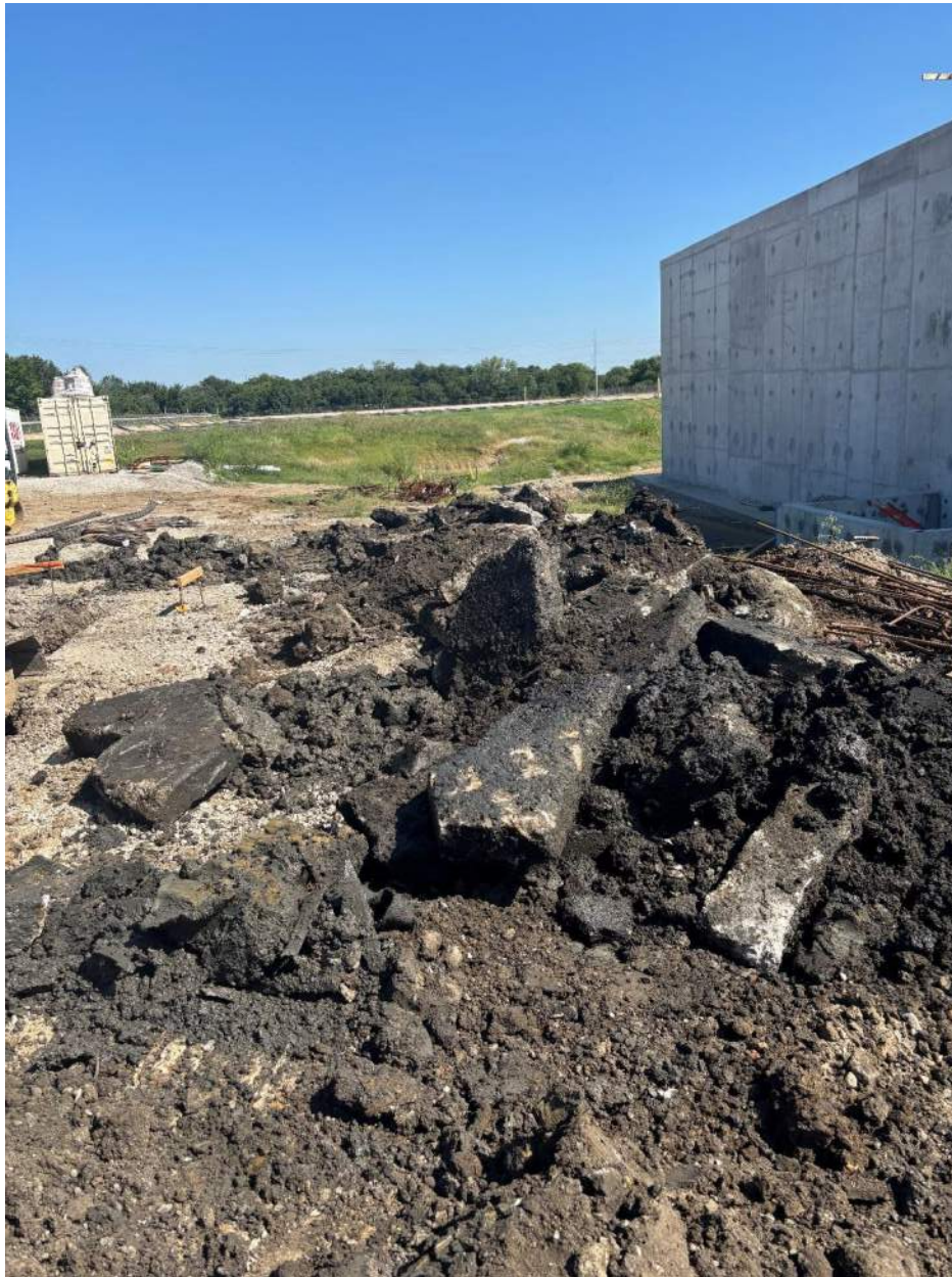
Photograph 8: Concrete rubble removed from test pit excavation along east edge of building
