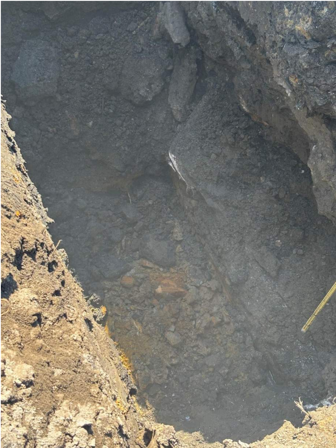
Photograph 11: Material change at NE to brown silty clay with highly weathered sandstone.
