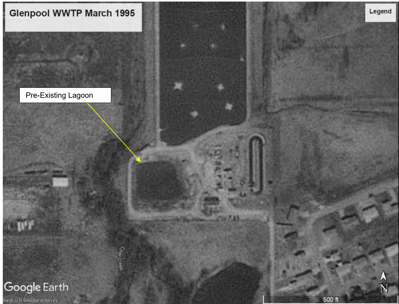
Figure 2: 1995 Google Earth Image of pre-existing lagoon
