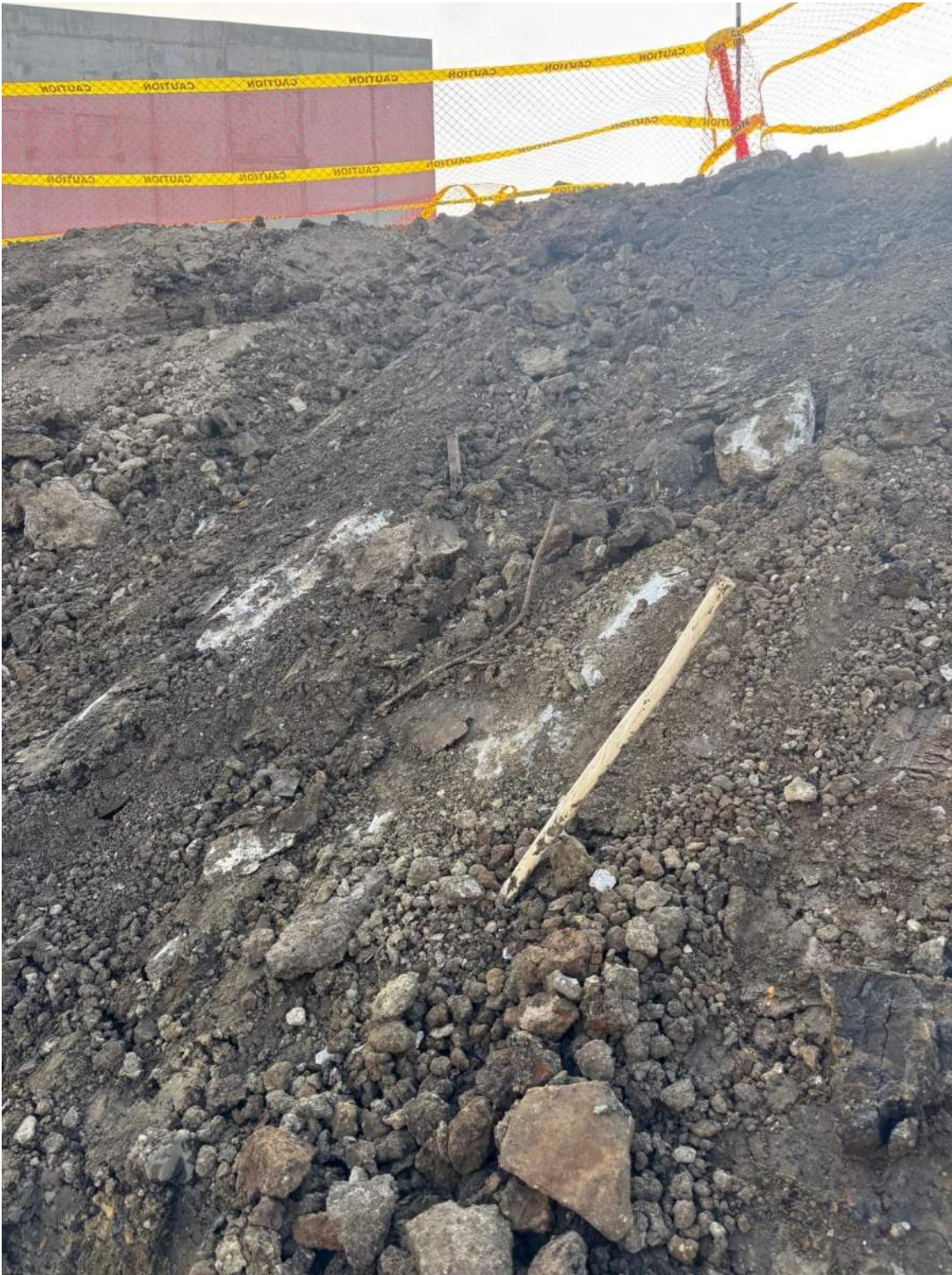
Photograph 3: Southeast corner of excavation with concrete debris in the sidewalls
