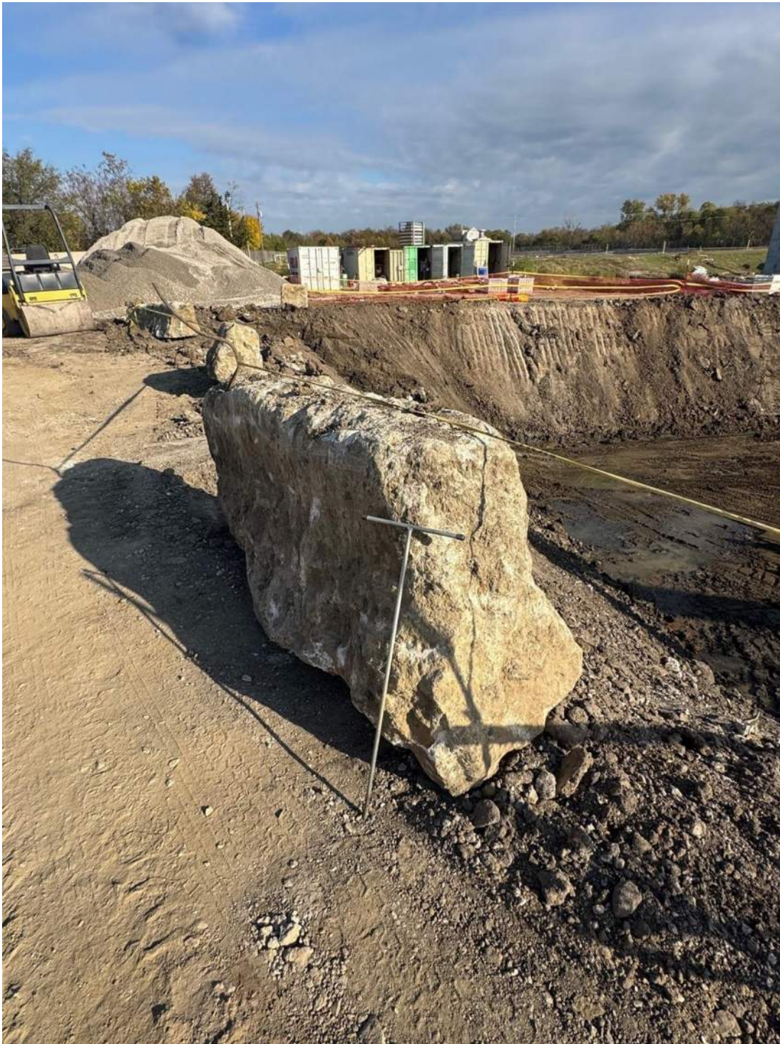
Photograph 5: Concrete block removed from excavation
