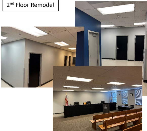
2 nd Floor Remodel
