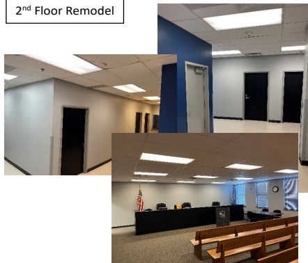
2 nd Floor Remodel
