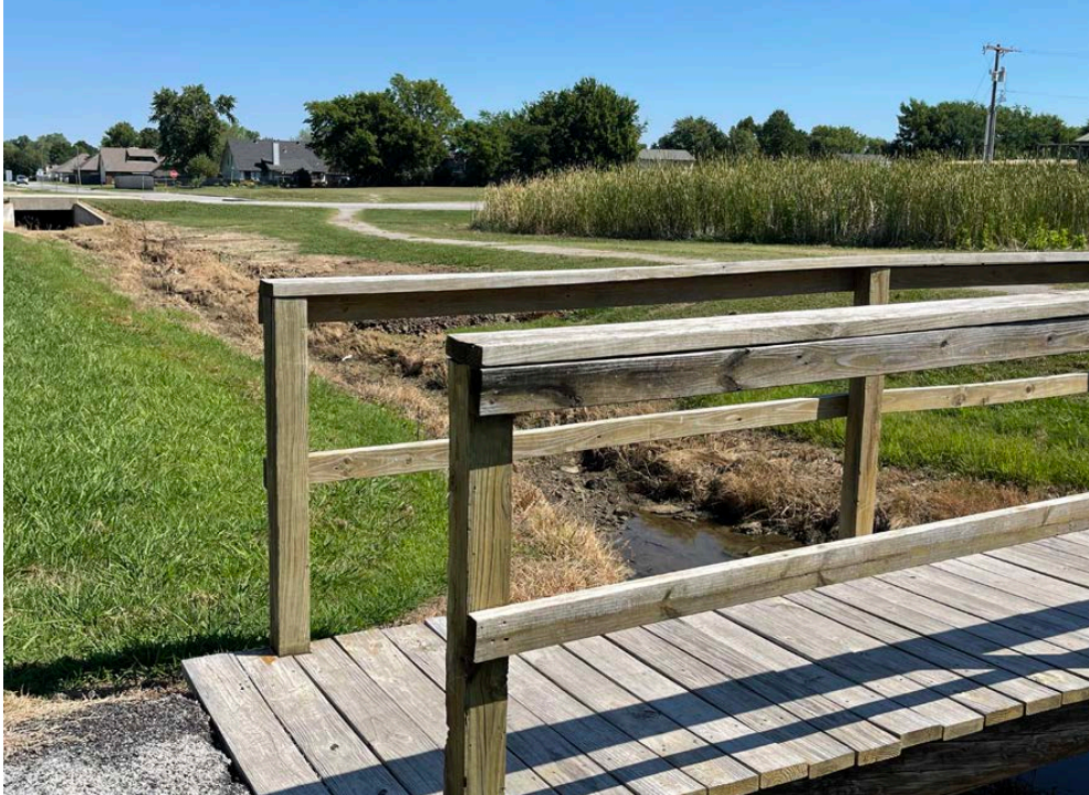
Existing dirt Sidewalk with wooden pedestrian bridge E. Warrior Road, 146 th St. -144 th Pl.
