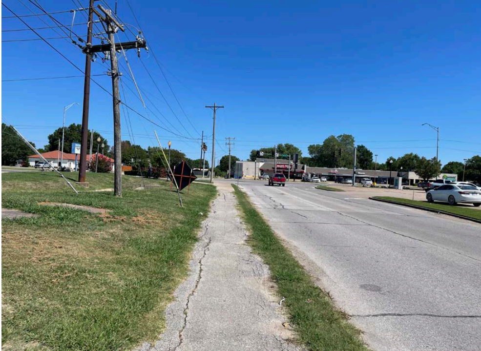
Existing Asphalt Sidewalk Eastside Warrior Road - 141 st .
