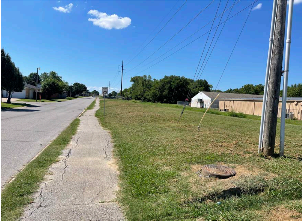
Existing Asphalt Sidewalk Eastside Warrior Road from 141 st – 146 th St.
