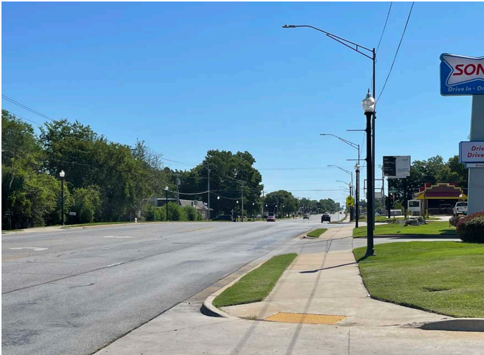
E. 141st Street showing ADA Sidewalk and Sign.
