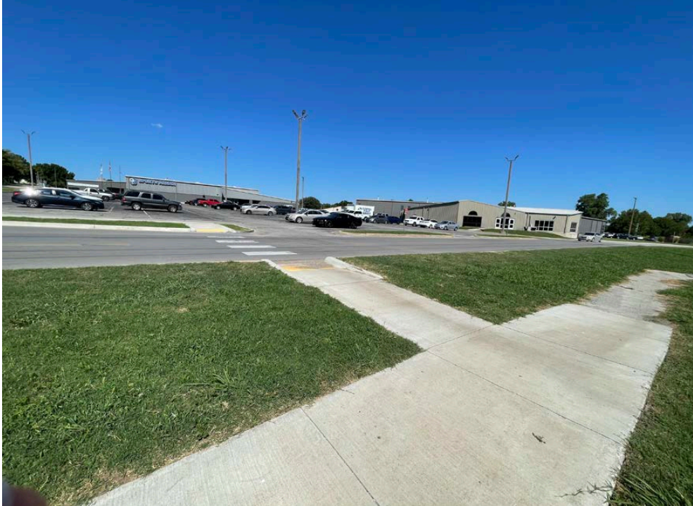
Existing ADA Sidewalk showing crosswalk striping. End of Existing Sidewalk at 146 th St. N. Warrior Road.
