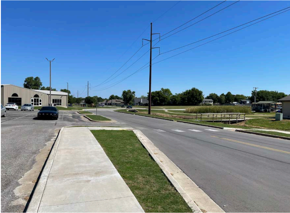
End of Existing Sidewalk from 151 st – 146 th N. Warrior Road.
