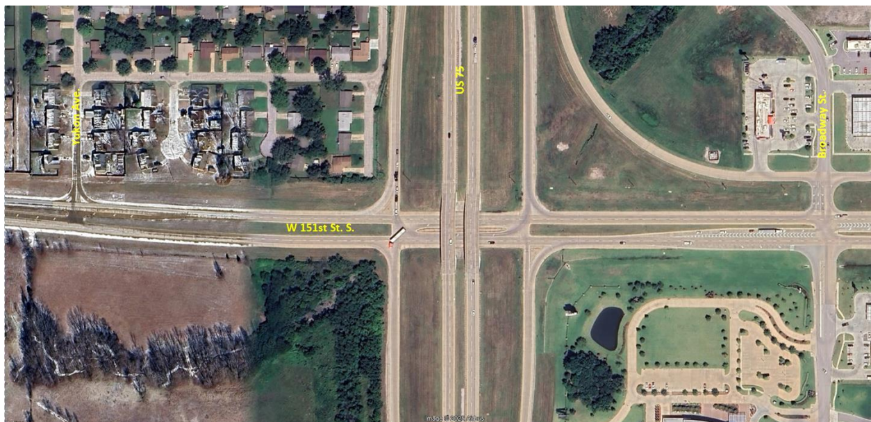
Figure 1. Existing Conditions – W. 151 st St. S. – Yukon Ave. to Broadway St.
