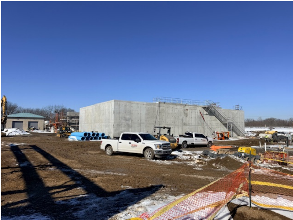
AEROBIC DIGESTERS
