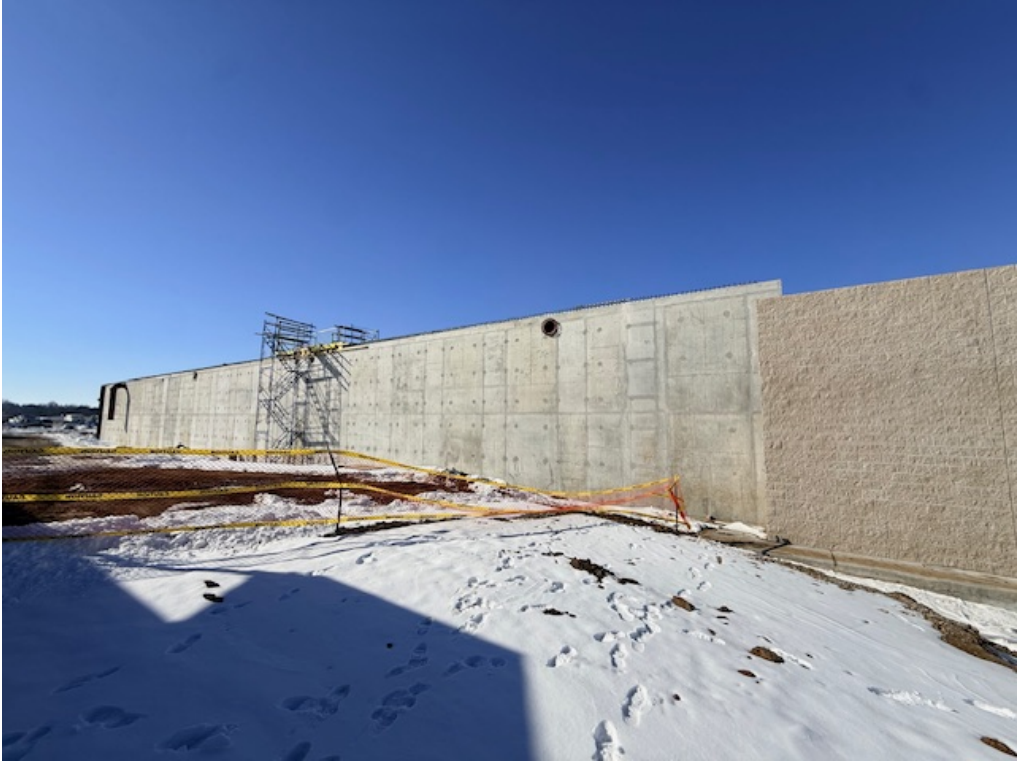
CONCRETE WORK ON THE SBR TANKS
