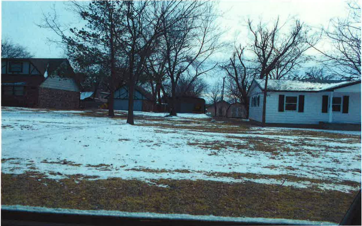
Subject tract: looking south from 147 th Street. (Shows relationship of carport to adjacent buildings.)
